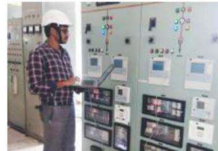
Retrofitting Works in 25 Substations in Himachal Pradesh
