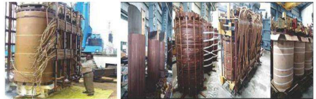
Power Transformers under overhauling & rewinding process
