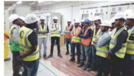
132/11kV Wakrah logistic -2 Substation
