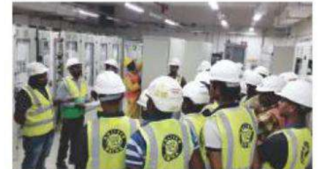
132/11kV Wakrah logistic -2 Substation
