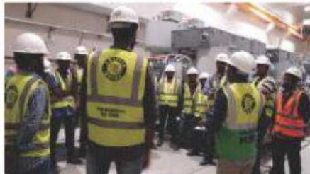
132/11kV Ras Abu Fontas-3 Substation
