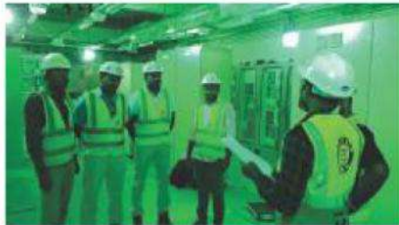
66/11kV Mehairja-1 S Substation
