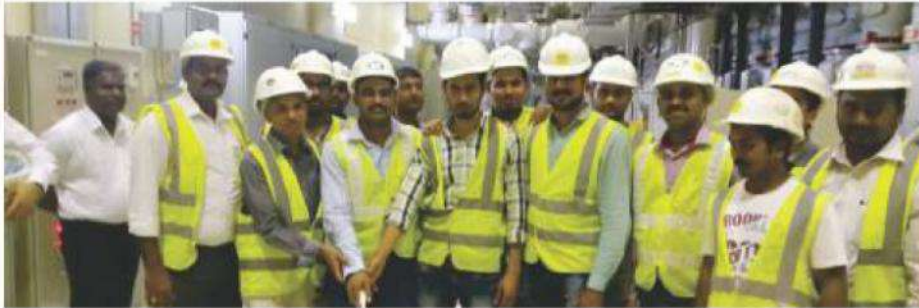
Successfully commissioned Phase 12 4Dohas substation
