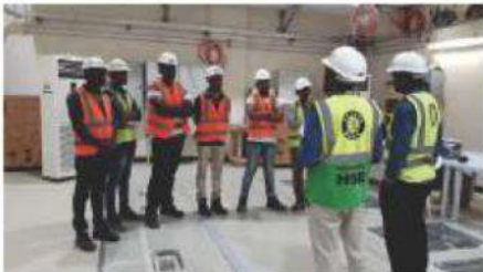
132/11kV Umm Al Hou1-2 Substation
