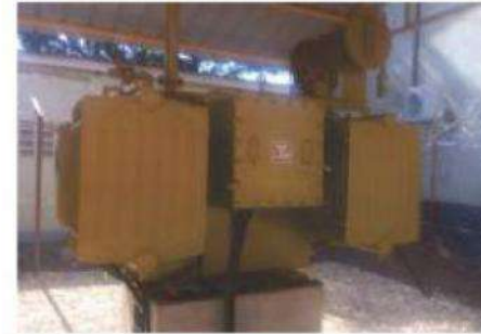
500KVA Transformer, 11KV Panel and LT Panels
